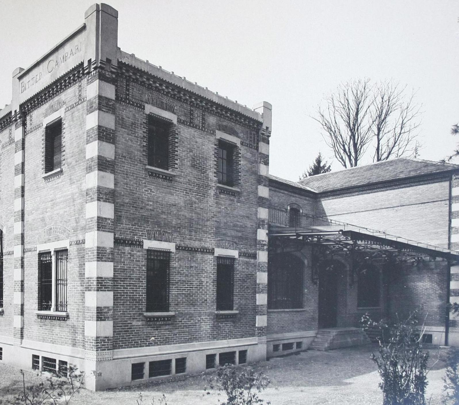
*Perrone responded to various particular production and plant-engineering requirements, unlike those of the metalworking and mechanical factories built in that period in the Sesto San Giovanni territory. In 1902, he therefore excluded plans for warehouses with sheds and designed a building capable of housing the entire production process. The layout of*
